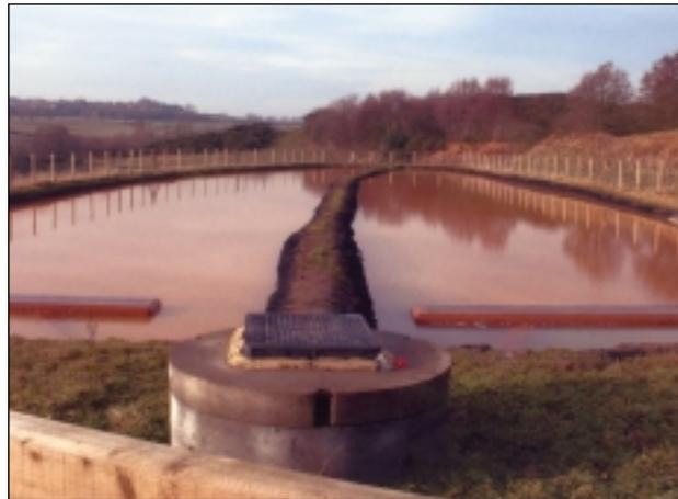
A number of monitoring boreholes into the workings had already been drilled by the Environment Agency to enable the rising minewater across the whole of the Colliery workings to be monitored. Initially the rate of rise of water in the workings was of the order of 9cm per day, indicating that urgent action would be necessary if a catastrophic polluting event was to be avoided.
